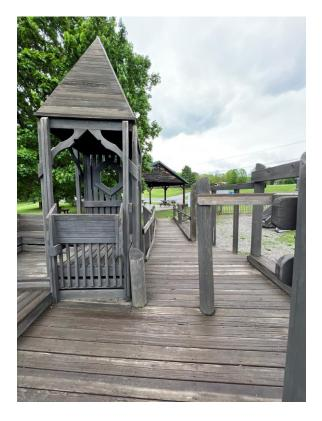
Fish Tunnel: Poor Condition Issues: The space between the post and baluster at the fish tunnel creates a head entrapment. (Priority 1). Space is over 3-1/2" and less than 9". Recommendation: Add filler pieces so spacing is less than 3-1/2".
